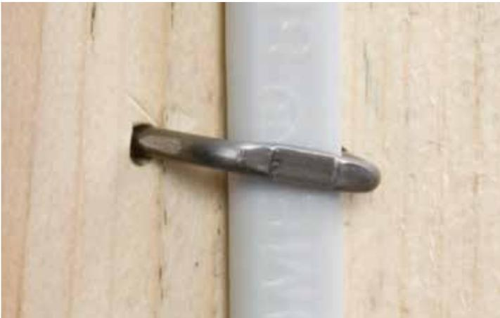
Photo 4: Example of potential line-to-ground arc fault (wire stapled too tight).
