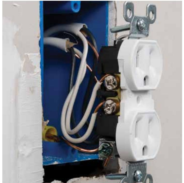
Photo 3: Example of series arc fault (pushing receptacle into box).
