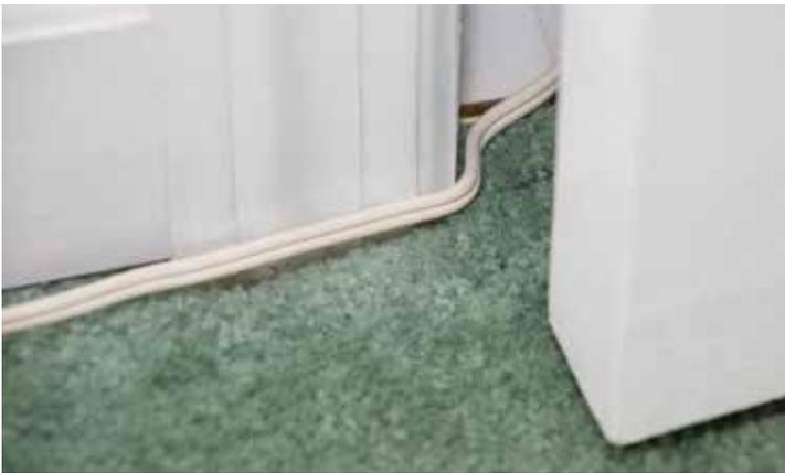
Photo 1: Example of line-to-neutral arc fault (door pinching power cord).
