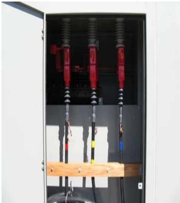
Picture 1 – BC Hydro Utility Service Cable Compartment
