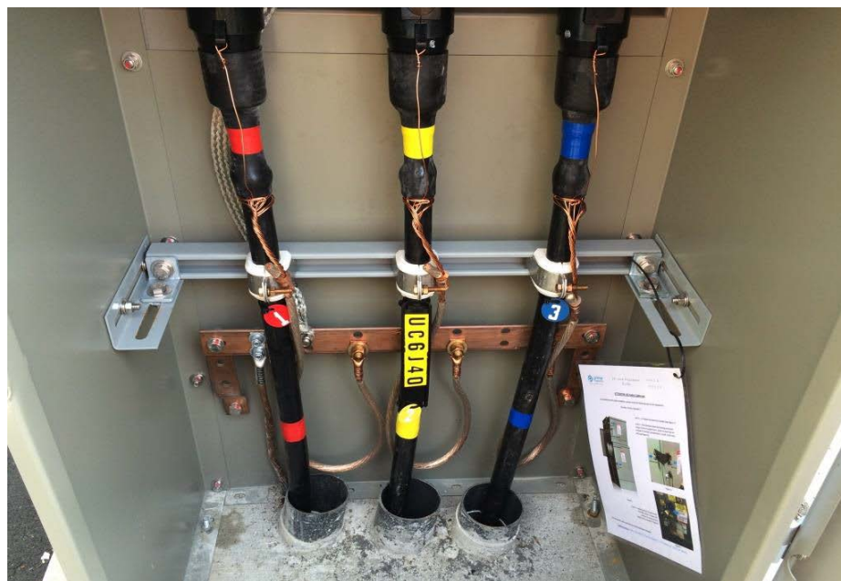
Picture 11 – Service Cable Clamps and Adjustable Cable Support Channel
