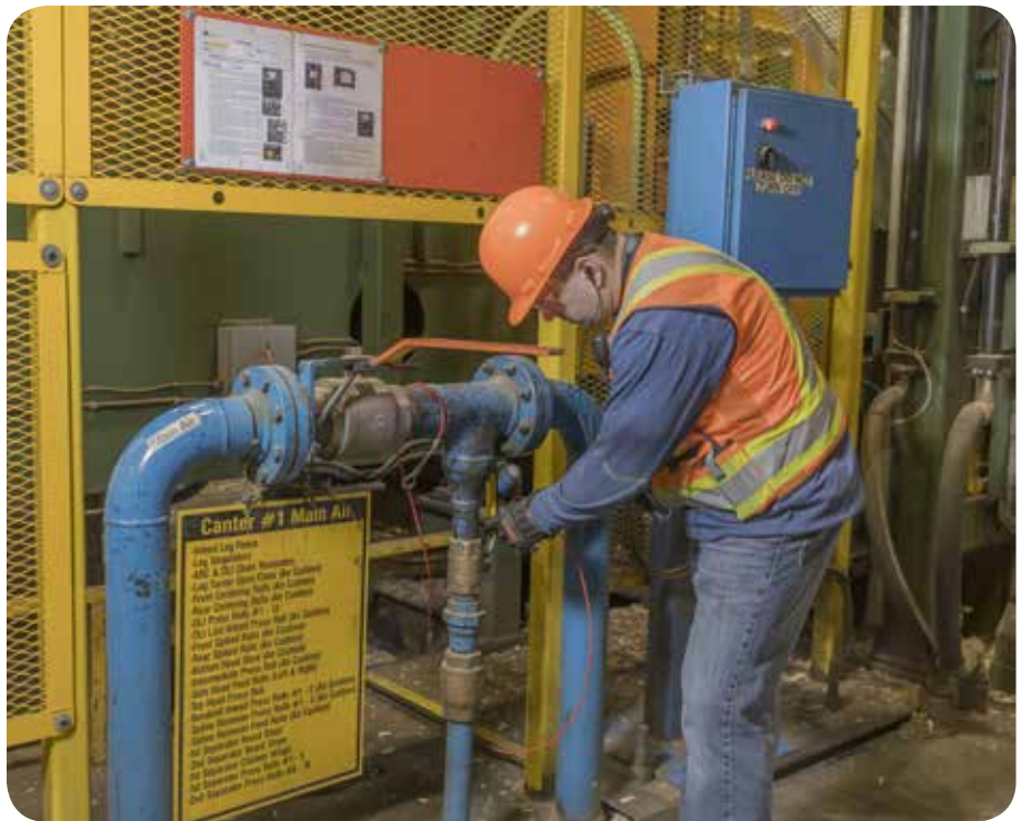
Figure 2: A worker performing lockout on a pneumatic (air) system.
