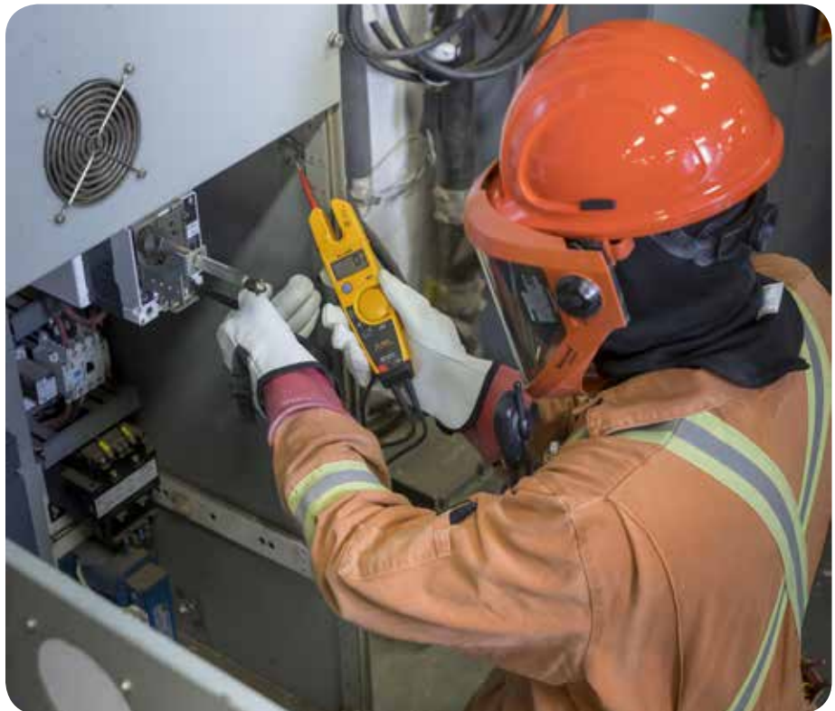
Figure 3: A worker with appropriate electrical arc flash protection.
