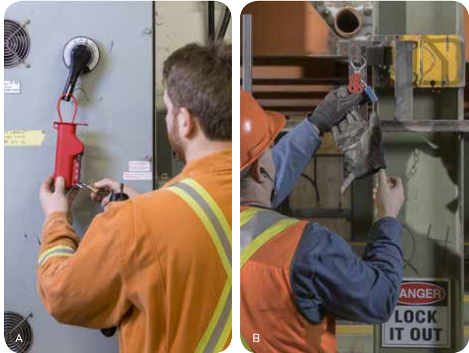
Figure 13: (A) A worker applying locks. (B) A worker applying a restraint pin.
