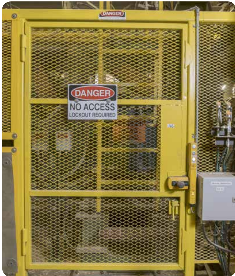
Figure 16: An electronic gate safeguard. The gate is controlled by the SRP/CS and will not open if the system detects energy or motion.
