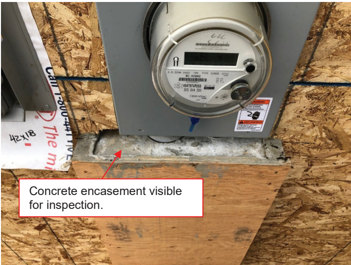
Figure 5. Option 2 with concrete encasement visible for inspection
