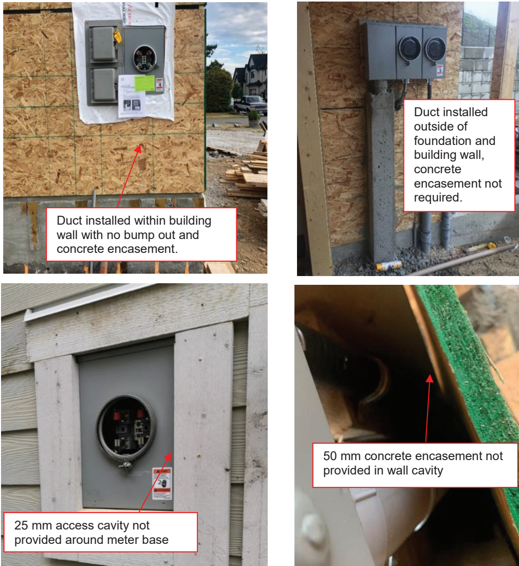
Figure 7. Non-compliant installations
